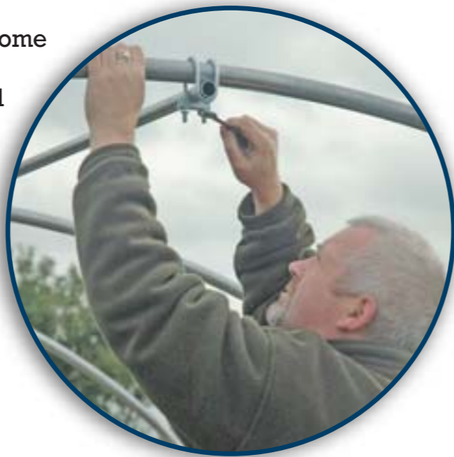
Above: Securing the overhead ridges to the hoop.
